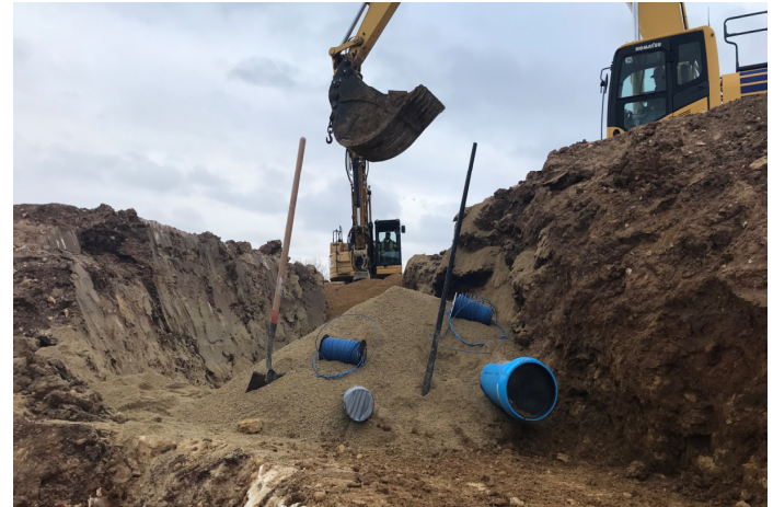
8" Fire & 4" Domestic Water Pipes (Southwest of Gym)
