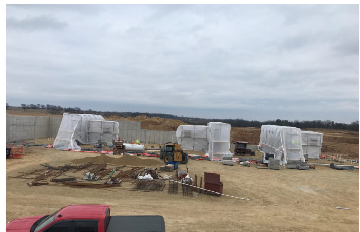
Masonry Hydro Set-Up (Locker Room Interior Masonry Walls)
