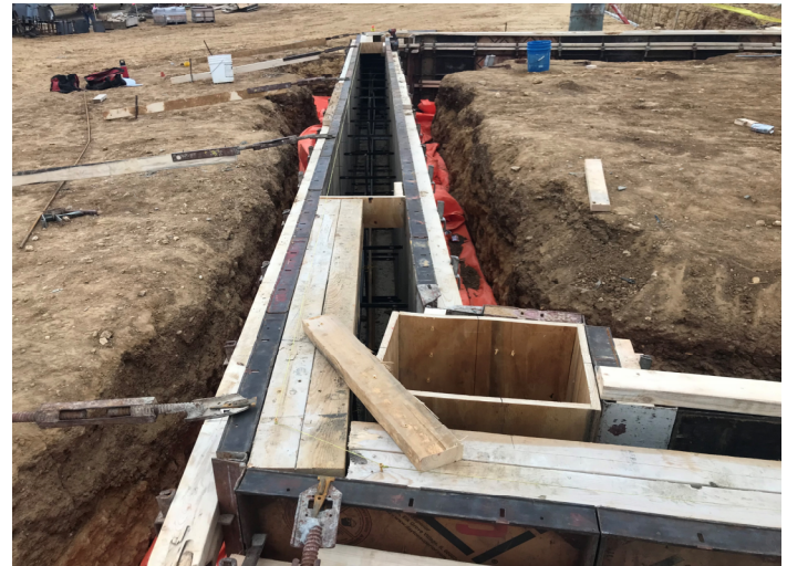
Forming and Pouring Concrete for Classroom and Commons Area Foundation Walls (NW of Building)
