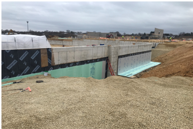
Waterproofing & Backfilling Gym Walls
